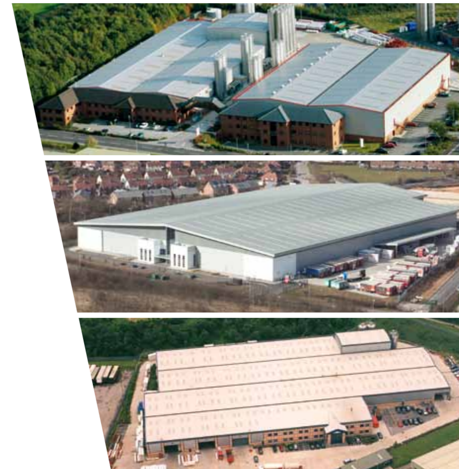
Our Derbyshire head office facilities, from top to bottom: 1) Main offices and extrusion centre 2) 25,000m 2 warehousing operations 3) Conservatory roofs and roofline extrusion facility
